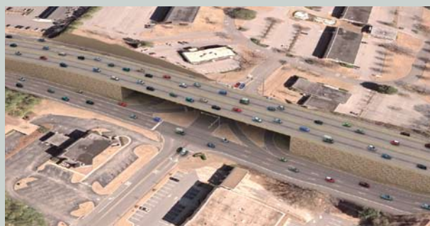
Grade separated intersection with US 280 crossing over cross street (rendering of Office Park Circle)
